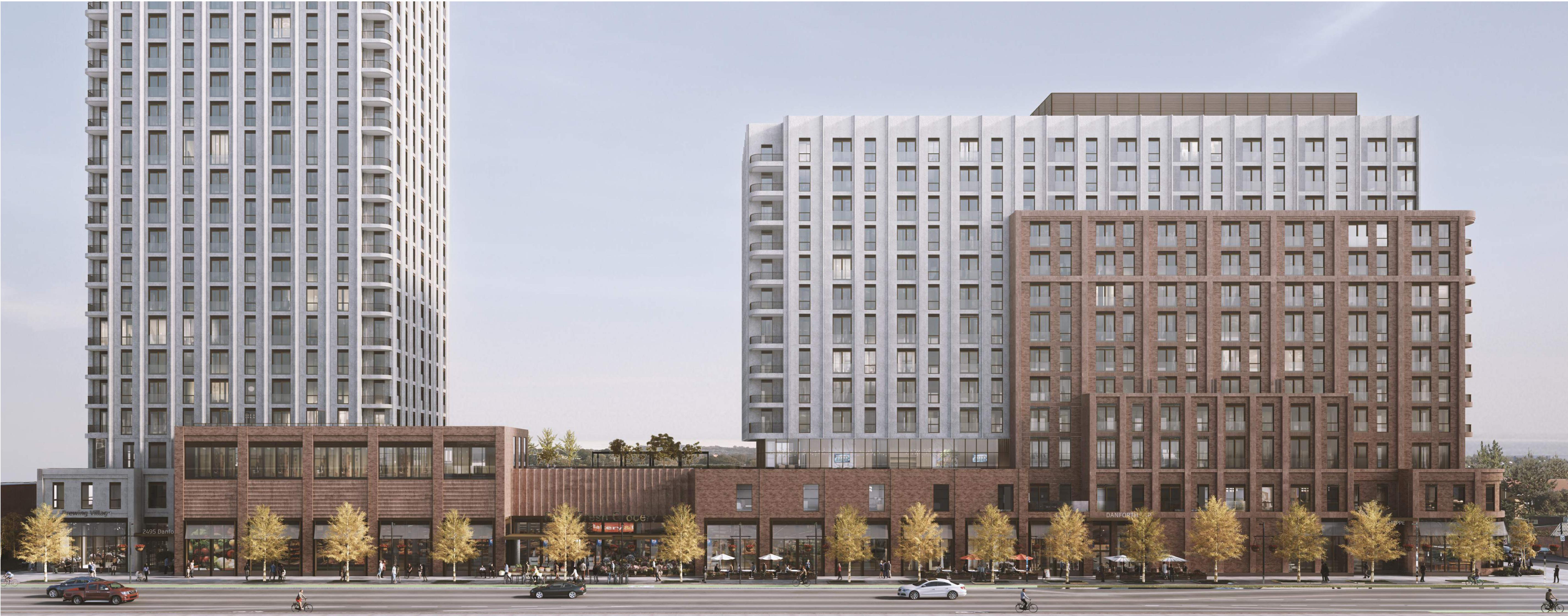
VIEW OF NORTH ELEVATION ON DANFORTH AVE
